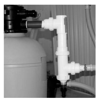
The UV Sterilizer is mounted directly to the filter using the threaded nipple provided
